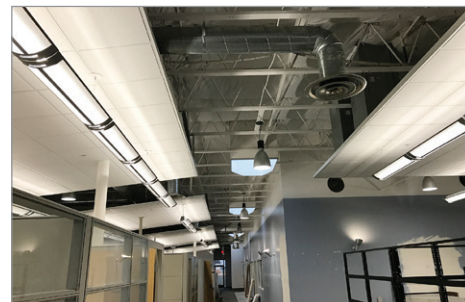
Construction at 6330 Hollister
